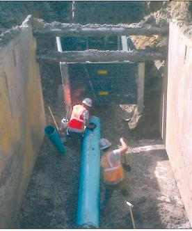
RIPA utilized a 4-sided modular aluminum Build-A-Box system from Efficiency Production to tightly shore around the installation of precast
