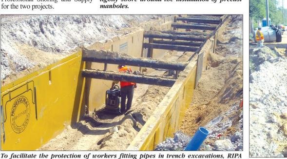
employed a series of Efficiency Production manufactured trench shields, also known as "trench boxes," to shore the pipelines. for the two projects.
